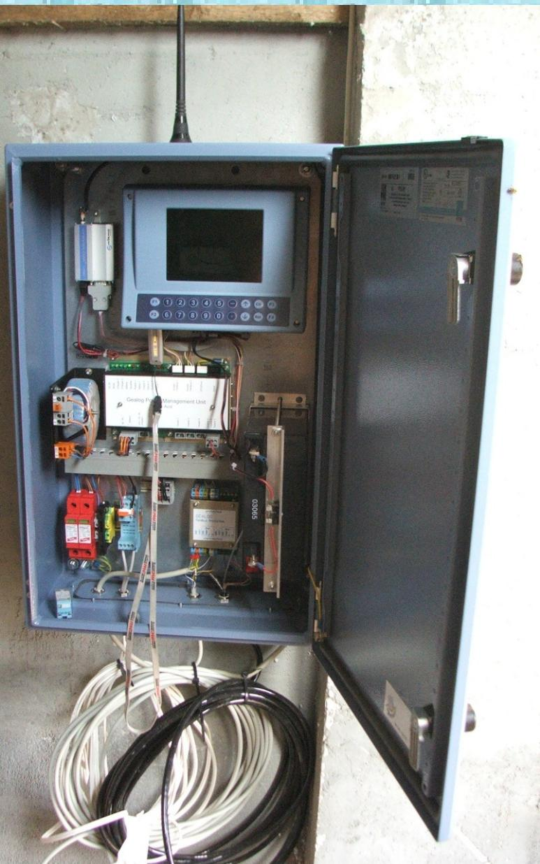
**Measurement equipment - YSI data loggers, powered from solar panels. GSM data transfer with mobile phone from stations to university PC.**
